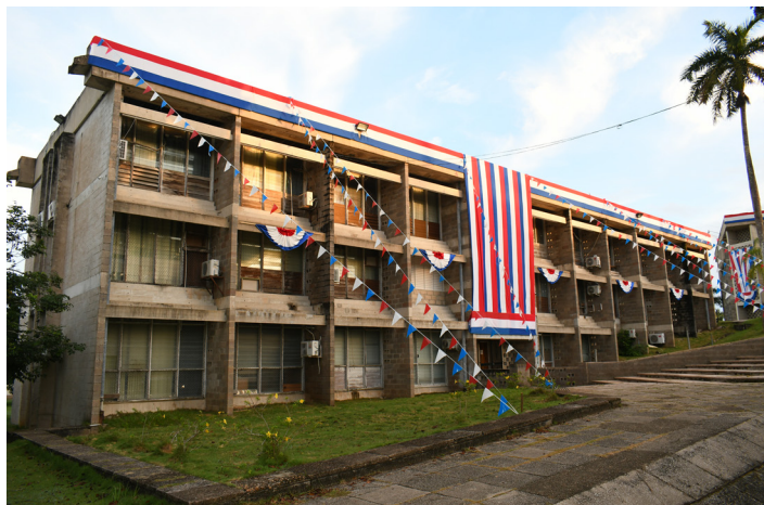
Headquarters of the MoECST at West Block, Independence Plaza
